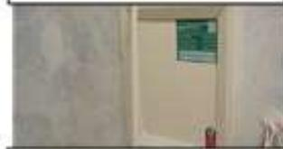
Asbestos panel to a riser at The Old Palace
